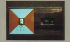
Fire extinguishers are mounted on all station platforms. Emergency telephones, indicated by a blue light, can be found near fire extinguishers in most stations.
